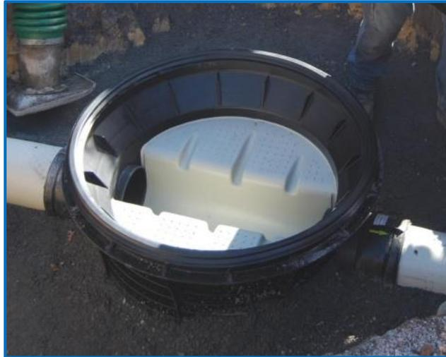
For all sockets horizontal angles of  $\pm 3.75^\circ$  or gradient changes up to 6.5% are possible. Direction and gradient changes at the same time will reduce the indicated maximum values accordingly.
