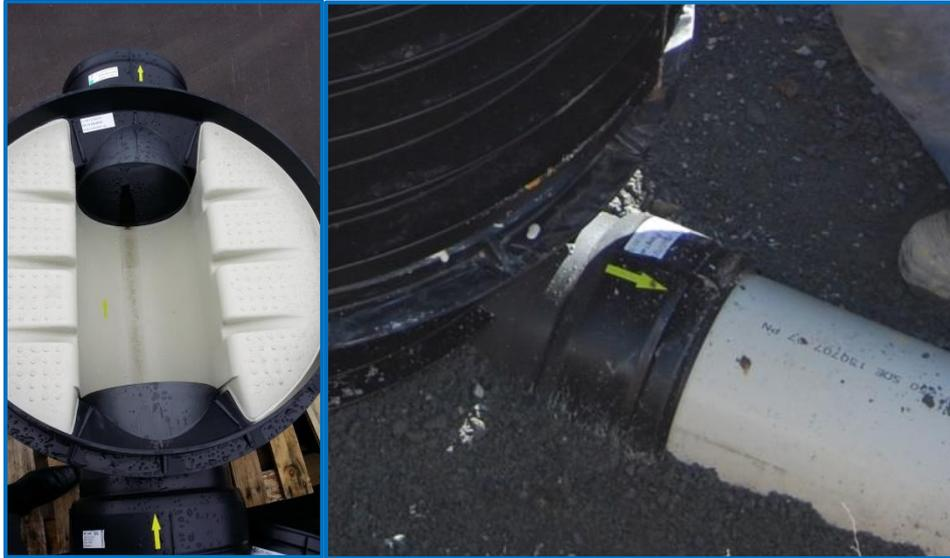
The Base should be checked with a spirit level to ensure that it is sitting level on the bedding.
