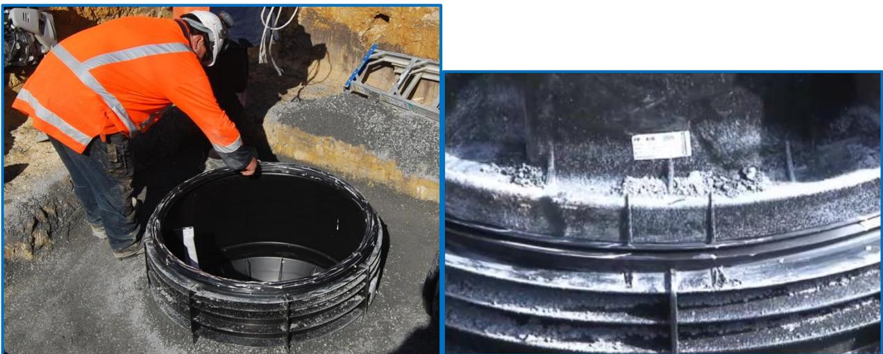
Align all manhole elements according vertical marks on the outside of the Riser and Cone elements to ensure the alignment of the ladder.
