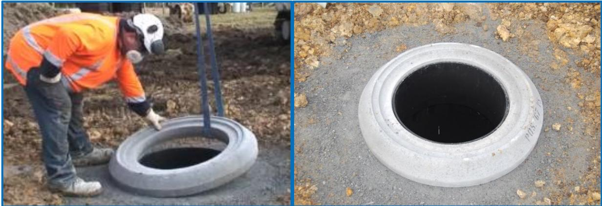
Below the LDR the bedding must be planar and free of point loads (consider using grit, sand or concrete dust). For class D applications, this should be prepared according to the design requirements for the road base course.
