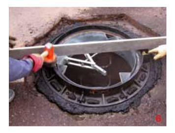
Check that the frame openings have been completely filled.
