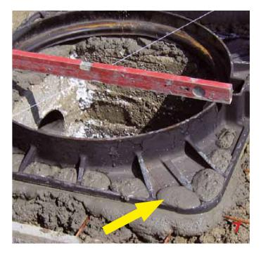
**8** Fill with sealing product. At this stage you may opt to vibrate the concrete using vibrating needles, providing that you ensure that this will not alter the level of the frame.
