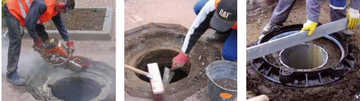
Check the diameter of the manhole opening or groove that the frame is to be fitted on.
